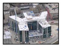
Installation of brick and metal panels continue on the exterior of the Critical Care Building.
